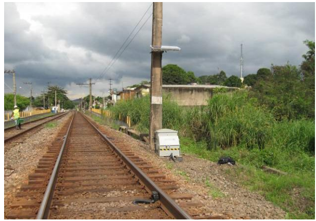
Figure 8: Typical installation of TOR unit.
